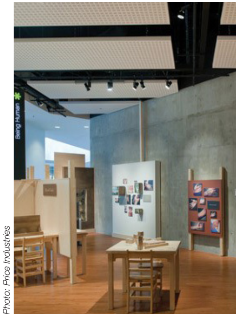
TELUS Spark Radiant Ceiling Panels
