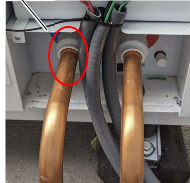
Connection between copper pipe and JG fitting
